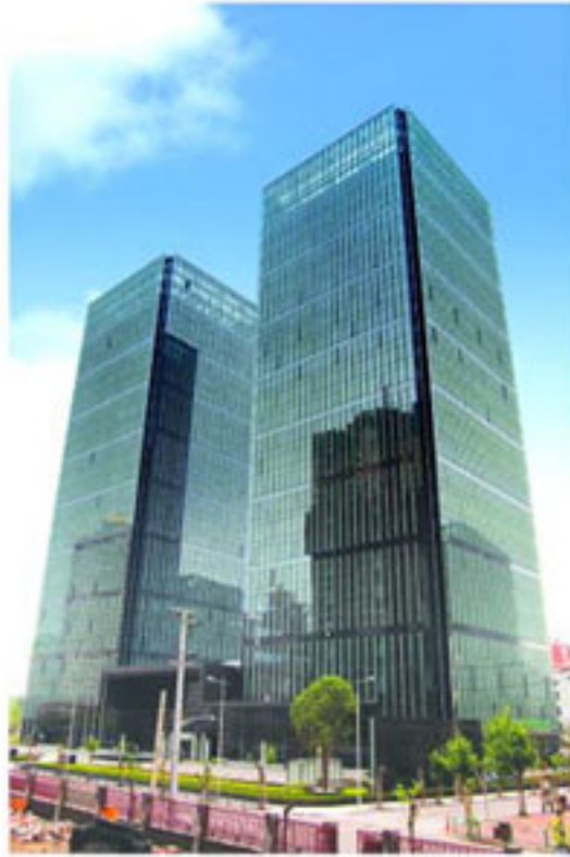
▲ Shanghai Eastern Tower
